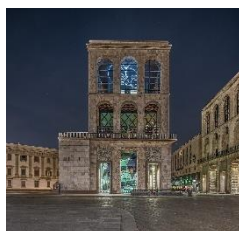
Fig. 4. façade revealing reactivated interior
