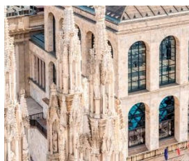
Fig. 10. historic structure and contemporary framing
